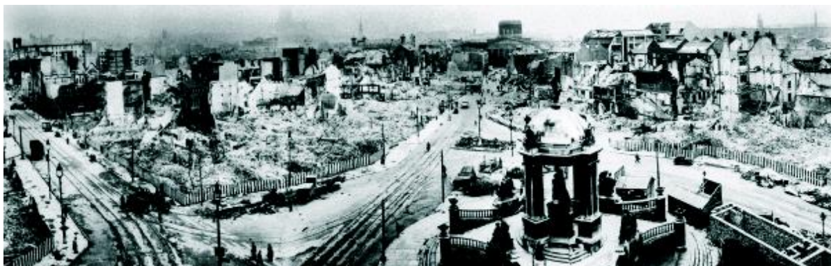
Devastation around the Victoria Monument 1944
